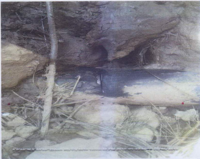
INCIDENT POINT AFTER EXCAVATION
