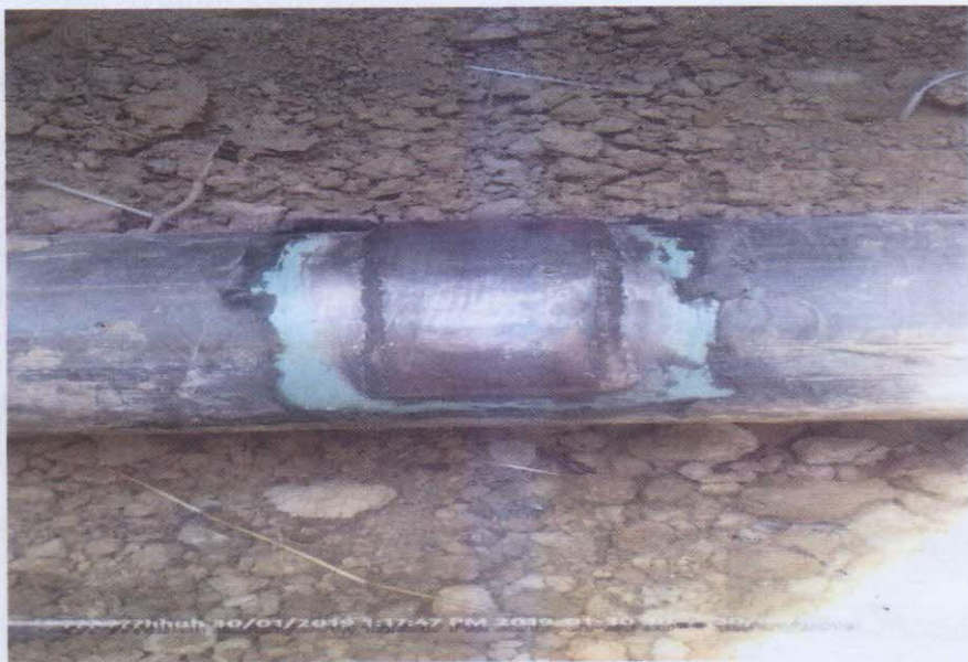
INCIDENT POINT AFTER REPAIR
